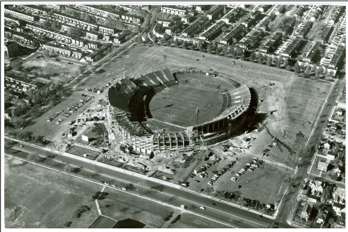
1953 Renovation and upper deck construction of Memorial Stadium 1
